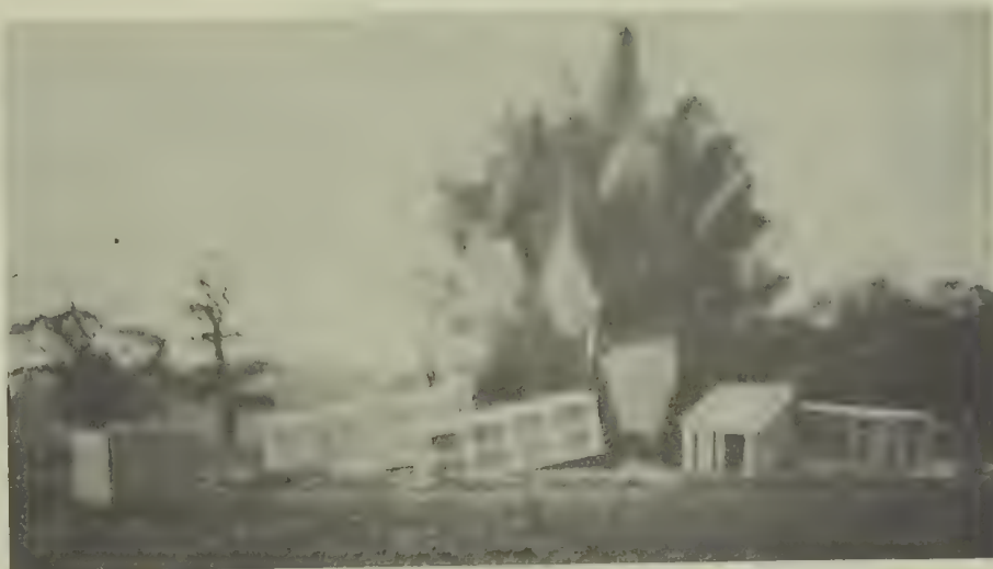
Fig.8.7 Effect of ground-shock on a group of reinforced brick surface shelters and one reinforced concrete shelter (on extreme left). Note how shelters are thrown into the air without fracture. (Paragraph 8)
